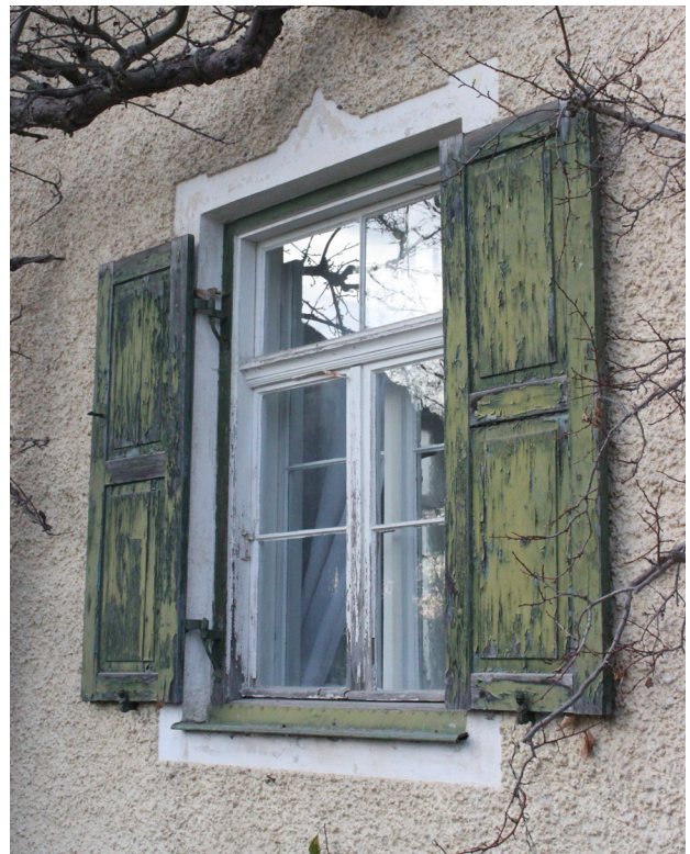
Abb. 7. Historisches Kastenfenster in Wessling, © Ralf Kilian, Fraunhofer IBP
